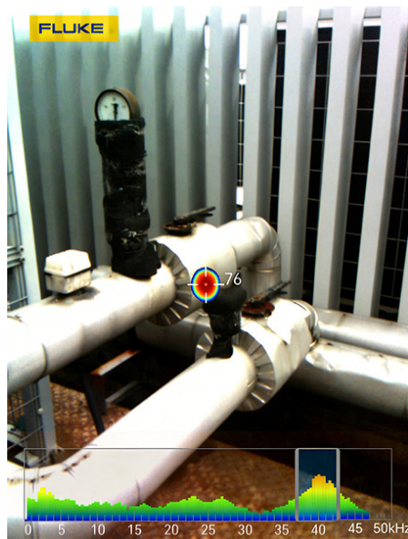
Leak detection on a pipeline
